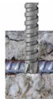
Rebar Step 2 Rebar Drill
