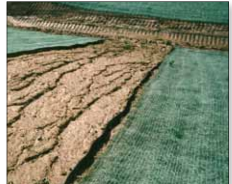
Green Curlex Blankets used in commercial slope application
