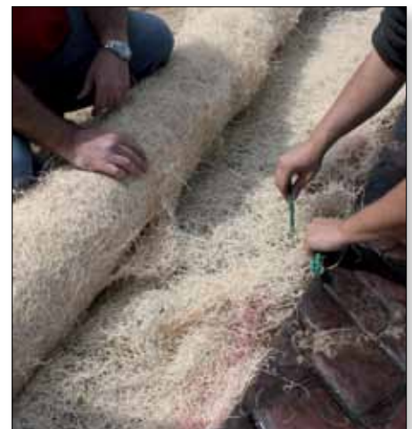
Install using DeWitt E-Staples
