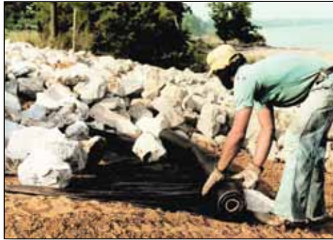
Filter Fabric application.
