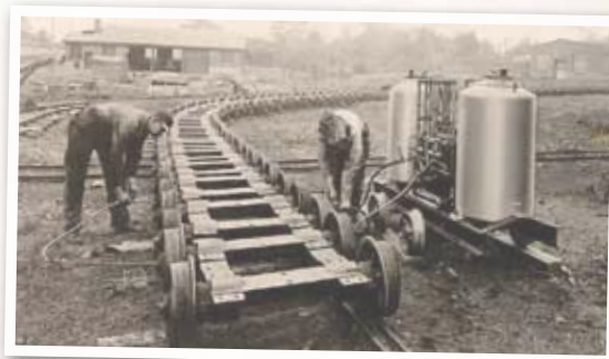
COAL CAR LUBRICATION SYSTEM
