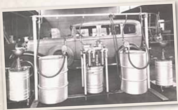
AN EARLY 1900'S LINCOLN® LUBRICATION SYSTEM
