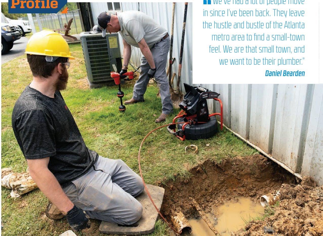
▲ Cody Letner, left, operates a RIDGID SeeSnake Compact C40 Reel and CS6X Versa Monitor camera, while Daniel Bearden uses a NaviTrack Scout Locator to see what they could discover for a business that was having a drain clogging issue.
