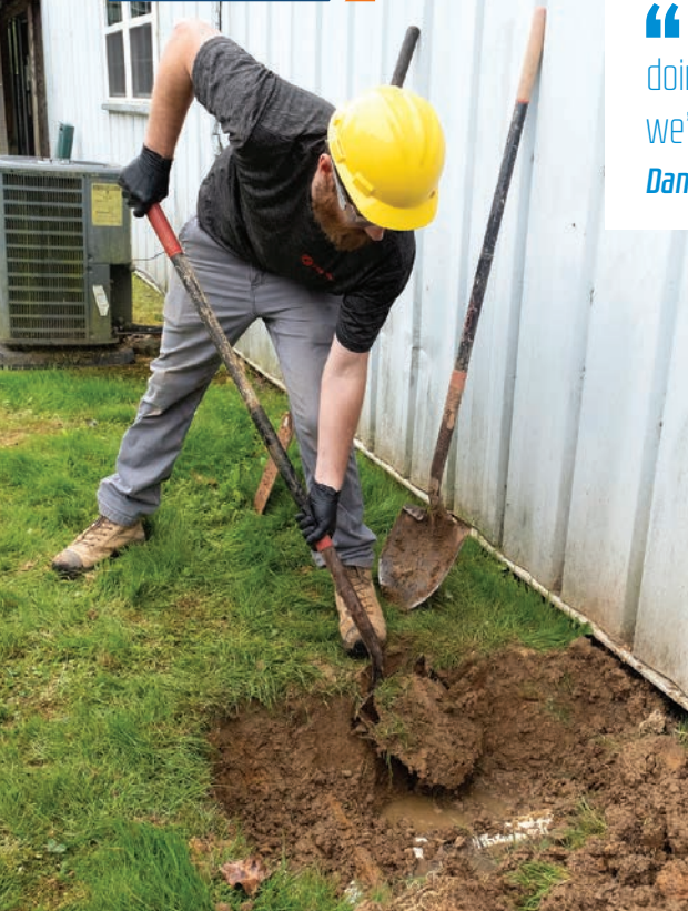
▲ Cody Letner digs to the pipe in order to run a camera inspection on it at a business job site.
