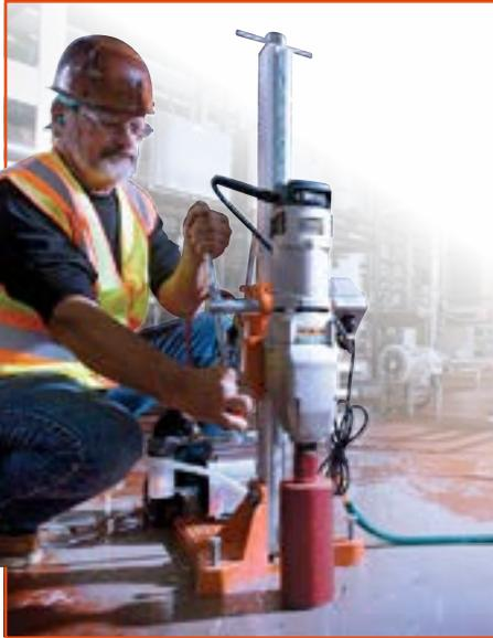
Core bits are cutting tools used to remove a cylindrically shaped piece of material. A core drill is designed to cut a hole and remove a core sample or to drill a hole without leaving material behind. Diamond core bits have diamond cutting tips and are frequently used for drilling in materials such as concrete, stone, and asphalt.
