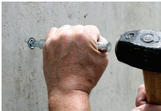
Anchor being set with hand setting tool.
