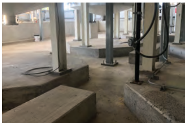
Typical medium-corrosive environment — exterior anchorage.
