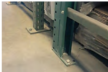
Typical low-corrosive environment — interior warehouse.
