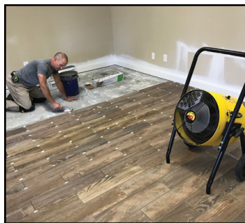
Pole Building / Workshop
