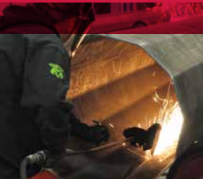
Weld removal with Tiger combo wheel.
