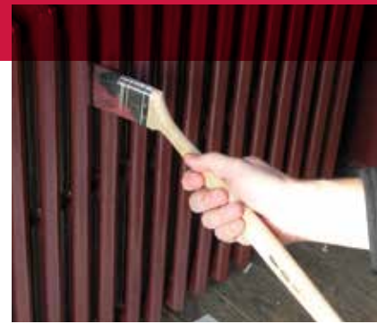
Painting inside the fins of a radiator with a Radiator brush.
