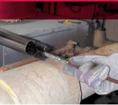
Cleaning boiler pipes with a flue brush.
