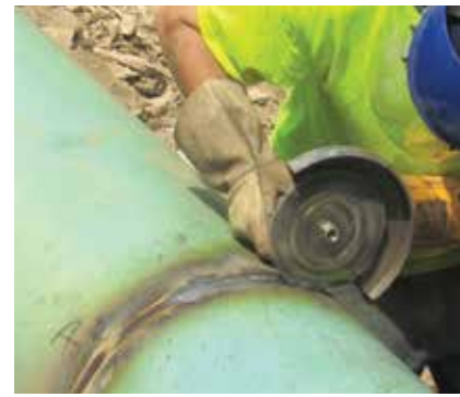
Removing weld slag before the next weld pass.
