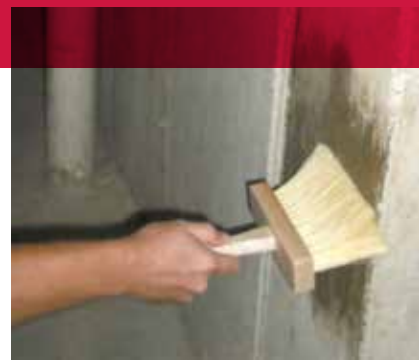
Applying waterproofing material with a masonry brush.
