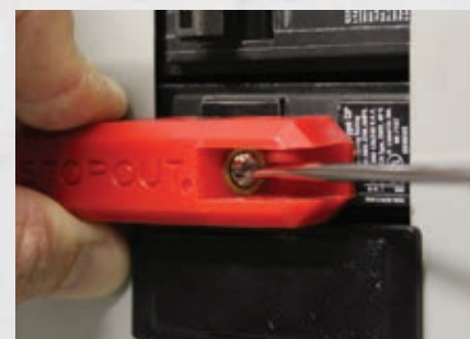
Tighten setscrew for secure fit.
