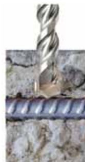
Rebar Step 1 Hammer Drill
