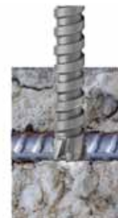
Rebar Step 2 Rebar Drill
