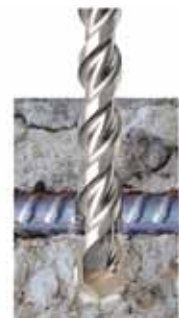
Rebar Step 3 Hammer Drill
