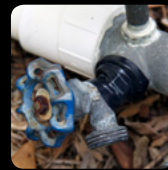
Repairs loose or leaky plumbing
