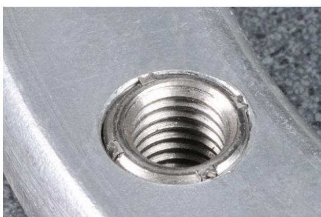
Correctly installed insert.
