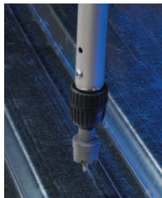
Drill Deck Holes
