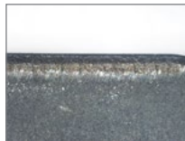
Thermal Cracks (Thermal Wear)
