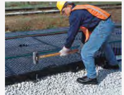
Side Pans are secured in place with 24" rebar fasteners. Typical installs require two pieces of rebar per Side Pan.
