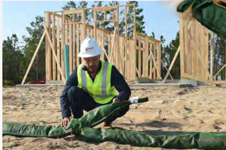
Use Sediment Removal socks for perimeter control on construction sites
