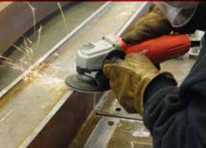
Smoothing the edges of roller coaster track with a resin fiber disc.
